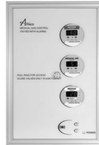
Alarm Valve Combo
